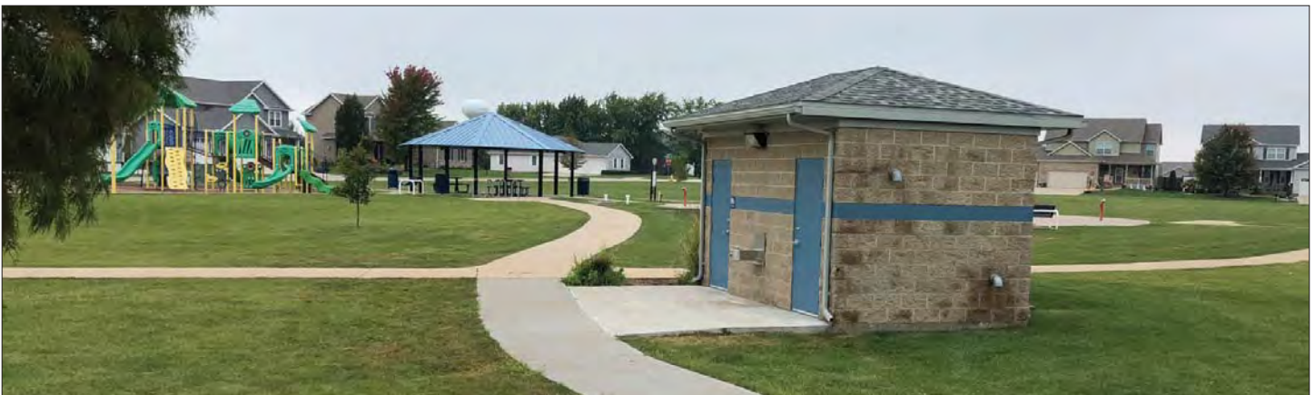
Permanent Restroom, Shelter, and 5-12 Play Structure
