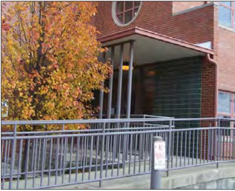
Accessible Southwest Entry
