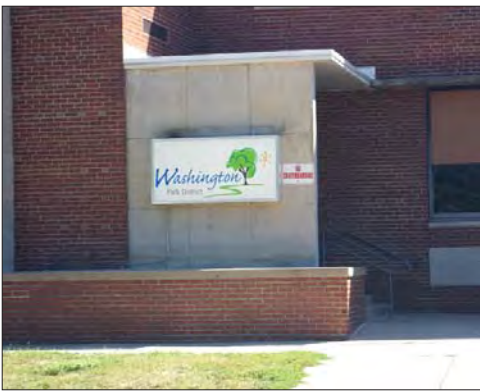
Entrance to Park District
