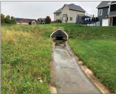
Detention Area with Concrete Channel
