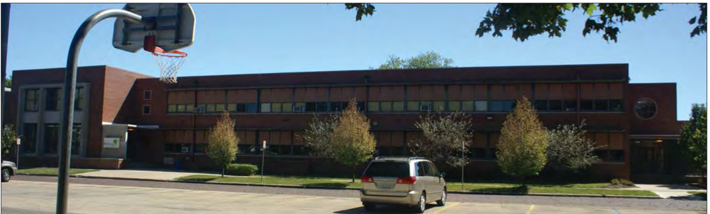
Spruce Street Facade
